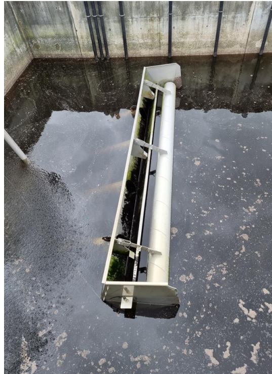
Settling/Decant mode* * Critical to retain the solids when decanting...
