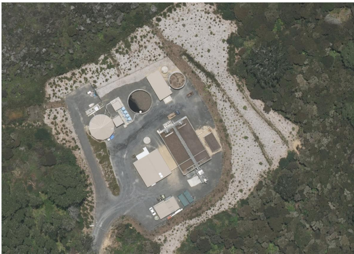
Figure 8-2: Mangawhai CWWTP layout (KDC Maps accessed 19/12/2023)
